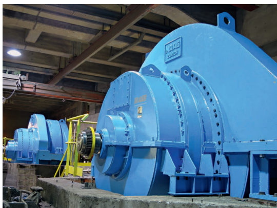
5 Completely reassembled and reactivated mill gear unit
